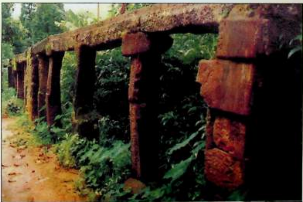
WATER CHANNEL (Śree Maha Viṣṇu temple, Thirunelly, Wayanād district)
