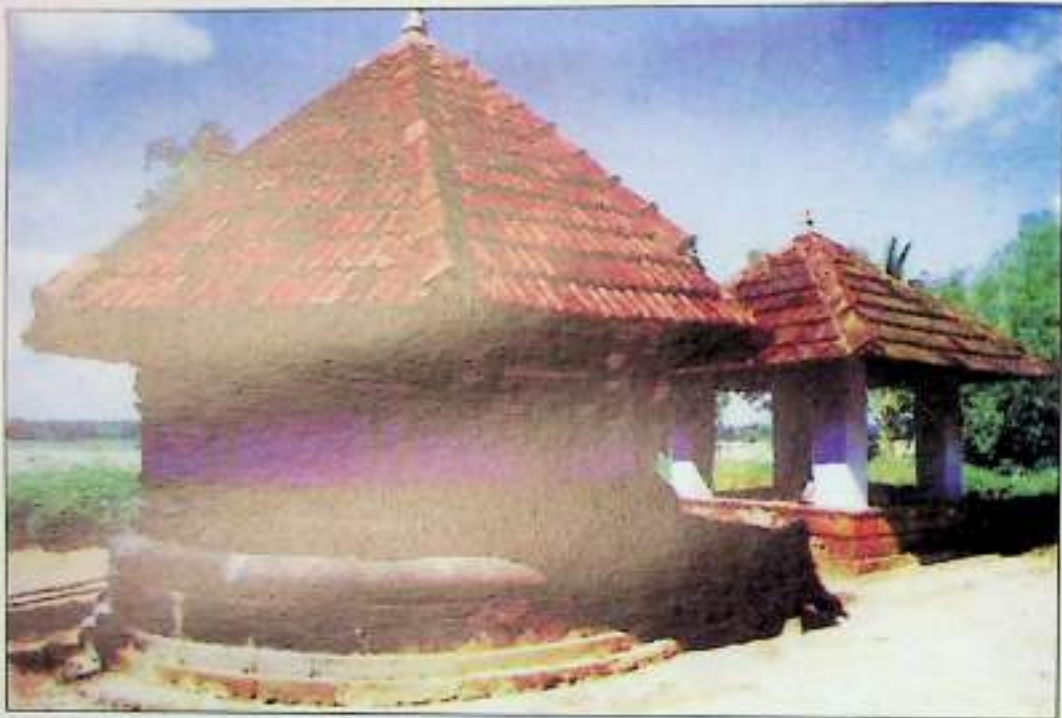
CIRCULAR ĒKA-THALA SREEKŌVIL WITH OCTAGONAL ROOF (Sree Brahma temple, Thavanoor, Malappuram district)
