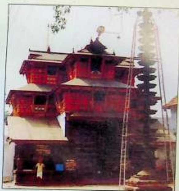
GÓPURA - TYPICAL KĒRALA STYLE (Eastern (front) gopura of Sree Poornathrayēsa temple, Thrippunithura, Erṅākulam district)
